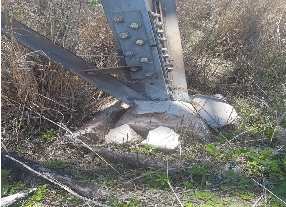
Figure 3: Broken foundation cap
