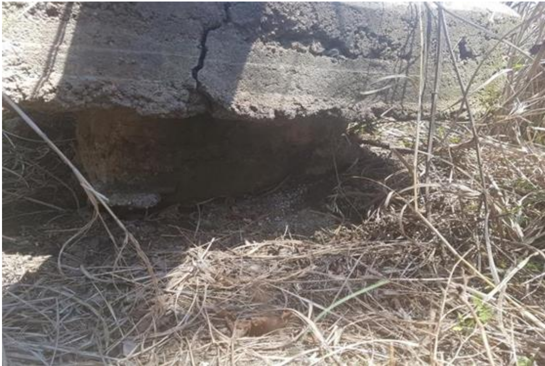
Figure 2: Soil erosion under the foundation
